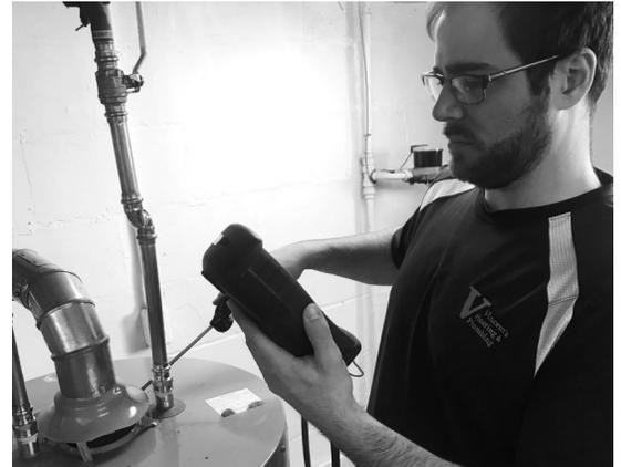
Here is Brendan performing combustion testing on a gas water heater to make certain it is performing as intended and not making too much carbon monoxide.
